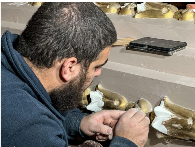
Restoration of the casework
